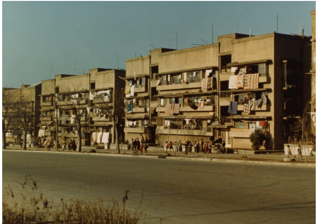
Tokyo apartment complex (ca. 1960s)
